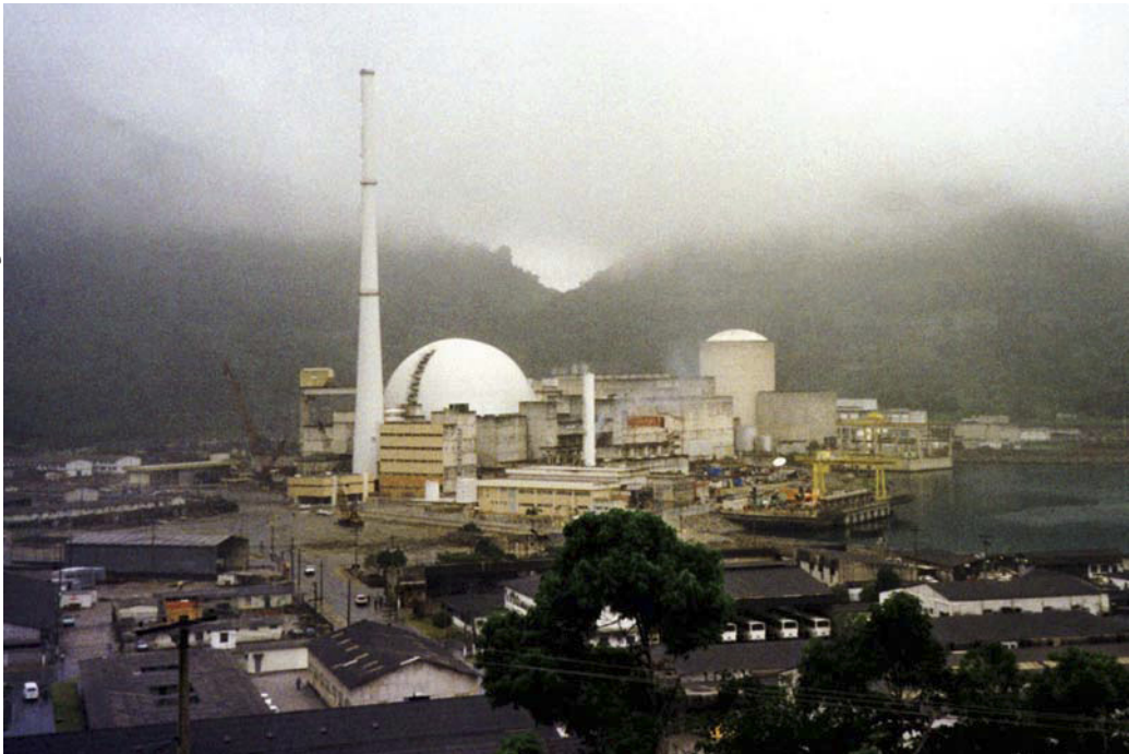
Almirante Álvaro Alberto Nuclear Center, in the surroundings of Angra dos Reis, Rio de Janeiro.
