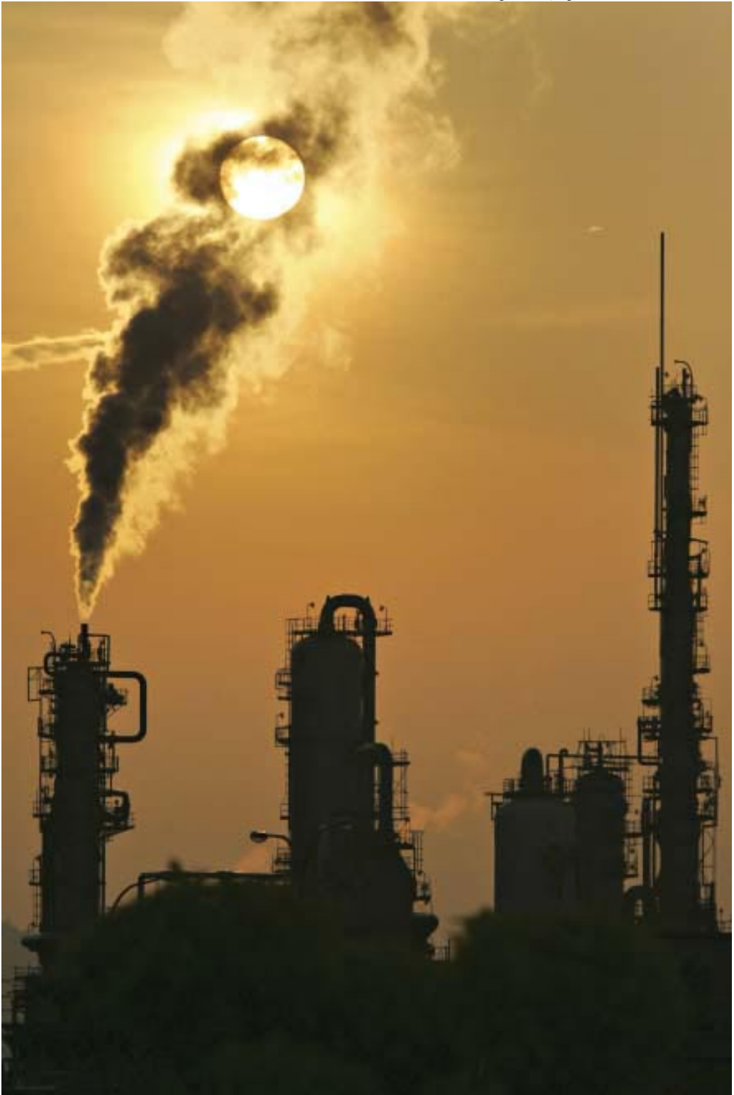
Chimney stack at the petrochemical complex in Paka, Terengganu State, Malaysia.
