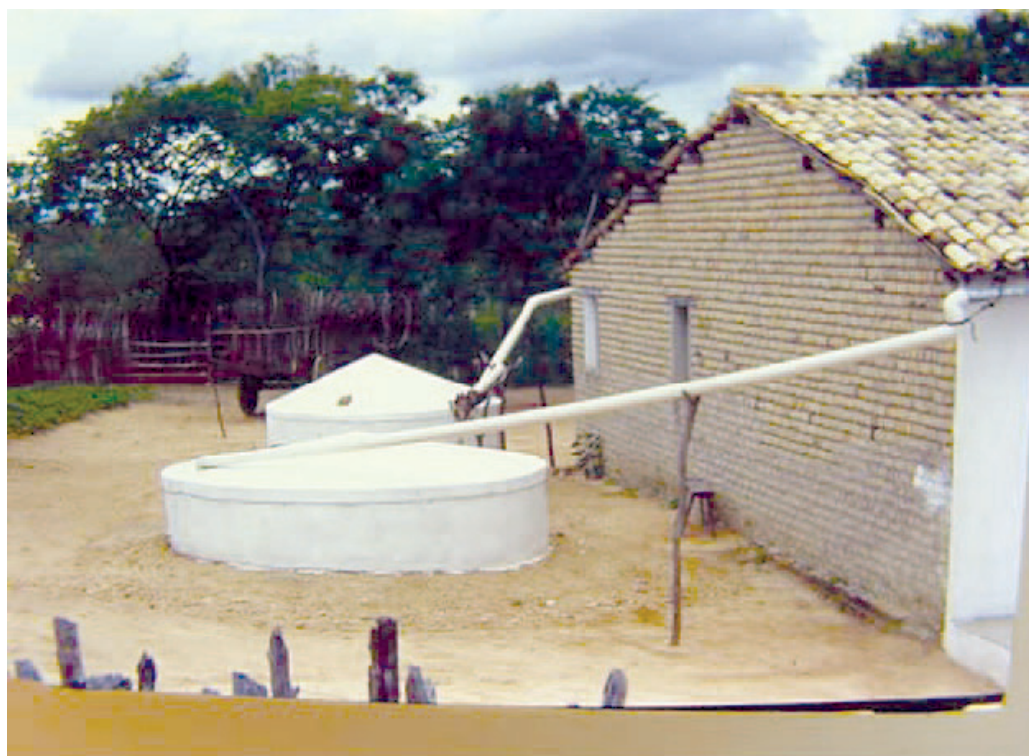
Figure 7 – Pane cisterns and the system of collecting water from the roof.
