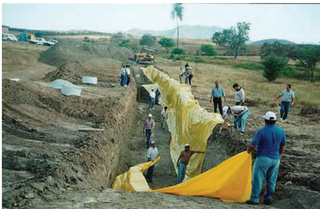
Figure 8 Construction of the underground dam – excavation and placement of the waterproof cover.
